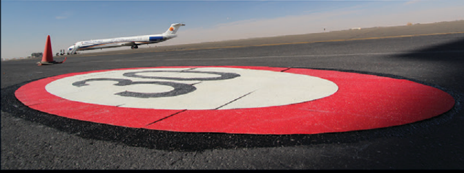
Service Road Marking
